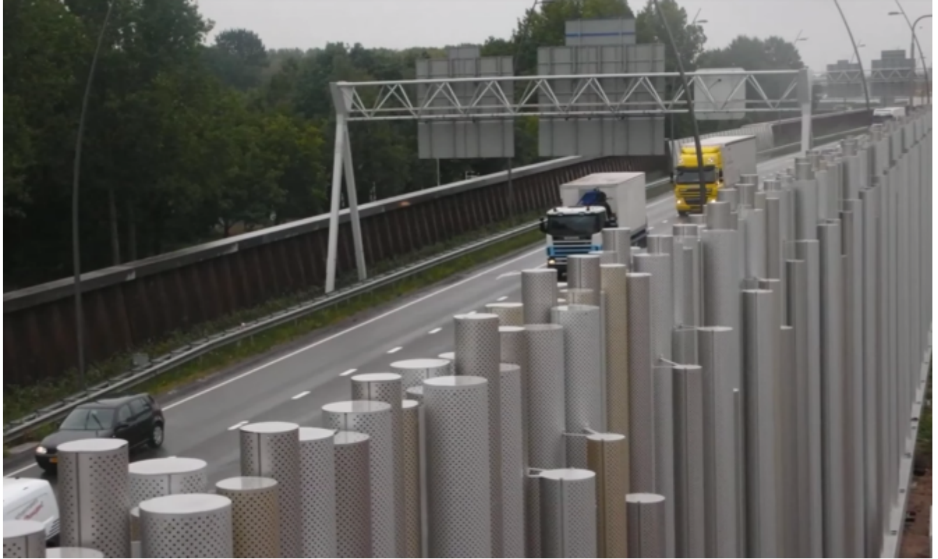
Figure 34 sonic crystals barrier at Netherland's Eindhoven A2 highway created by Van Campen Industries (source: https://youtu.be/lzNWC0scPTY visited on July 30th 2019 )
