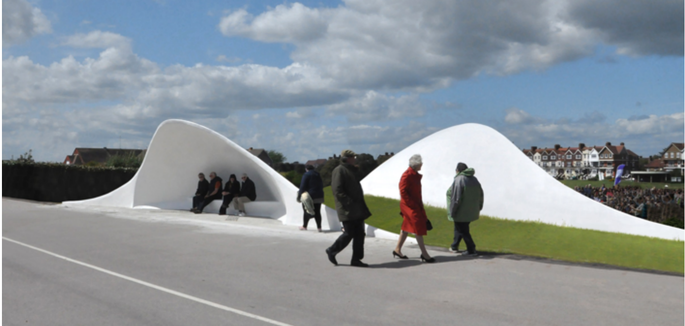
Figure 8 Flanagan Lawrence's acoustic shell in Littlehampton, West Sussex, UK, (Flanagan Lawrence, 2019)
