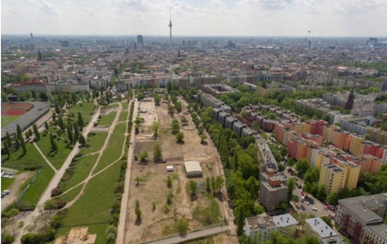
Figure 14 Mauerpark in 2017 with western part under construction, seen from a south oriented point of view, (Photo: https://gruen-berlin.de/projekt/mauerpark Visited on 30 th of July 2019)
